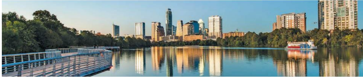
Boardwalk on Lady Bird Lake by Limbacher & Godfrey Architects Photo by Jeffrey P. Buehner
